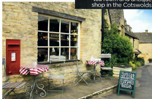
Guiting Power Post Office combines with an English tea room and antique shop in the Cotswolds
